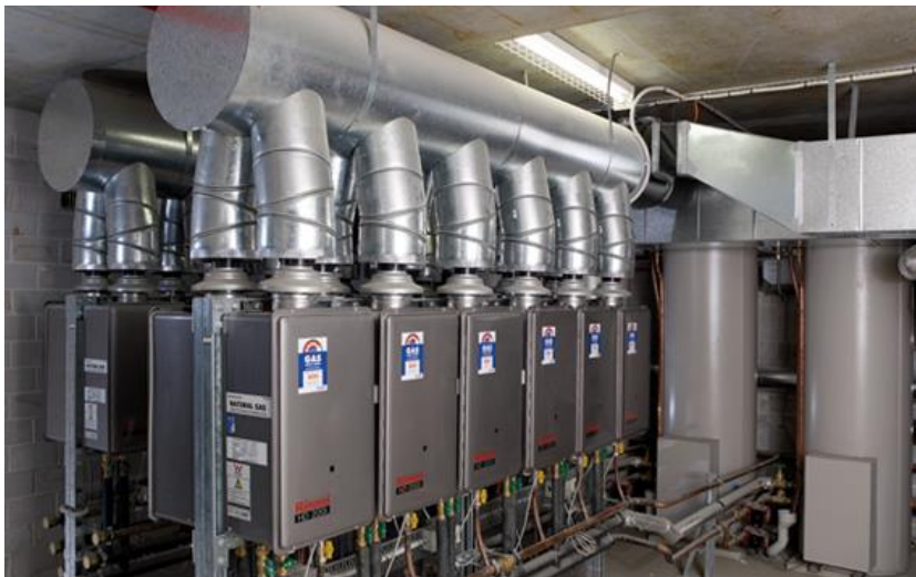
Figure 5: Typical multi-storey apartment block hot water system
